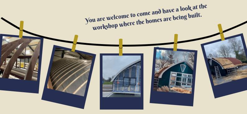
The houses are built smartly: the wall is constructed from CNC cut round trusses, which are placed with millimeter accuracy, then wall construction in 10 layers and always by means of bonding under pressure with stainless steel screws / nails.
